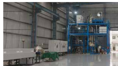
IAMP's facility under construction (Courtesy IAMP)
