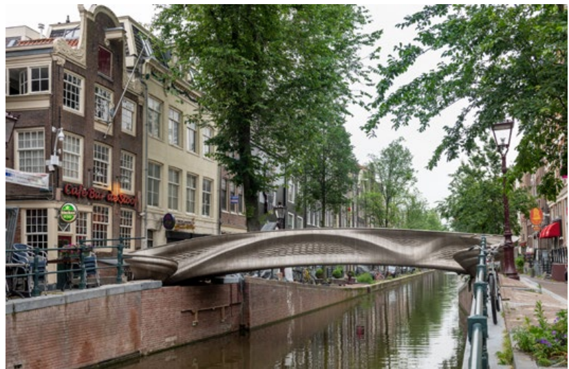
Fig. 6 The MX3D Bridge in its final form, installed and in public use as bicycle- and foot-bridge over the Oudezijds Achterburgwal canal. In a subsequent project, MX3D Smart Bridge, a sensor network was developed and installed in the bridge by The Alan Turing Institute to collect structural measurements such as strain, displacement and vibration, and environmental factors such as air quality and temperature, enabling engineers to measure the bridge's 'health' in real time and monitor how it changes over its lifespan. This data will also enable the bridge to 'understand' what is happening on it, how many people are crossing it, and at what speed (Courtesy MX3D)
