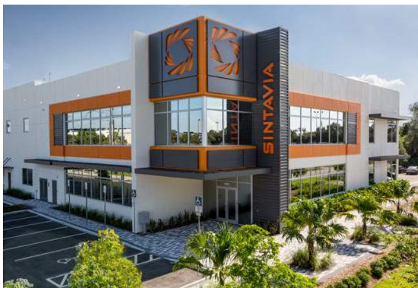
Fig. 1 Sintavia's new AM facility in Hollywood, Florida, USA
