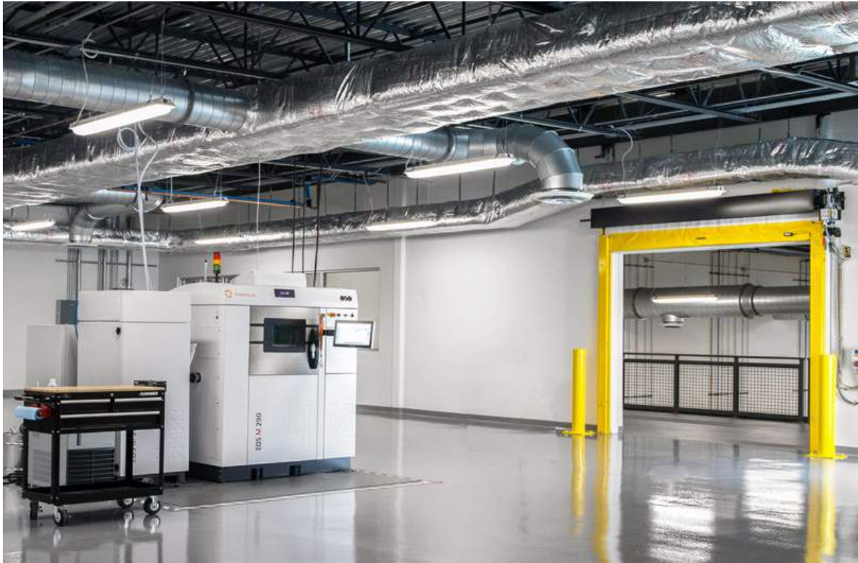
Fig. 8 One of five EOS M290 systems installed at Sintavia's new facility
