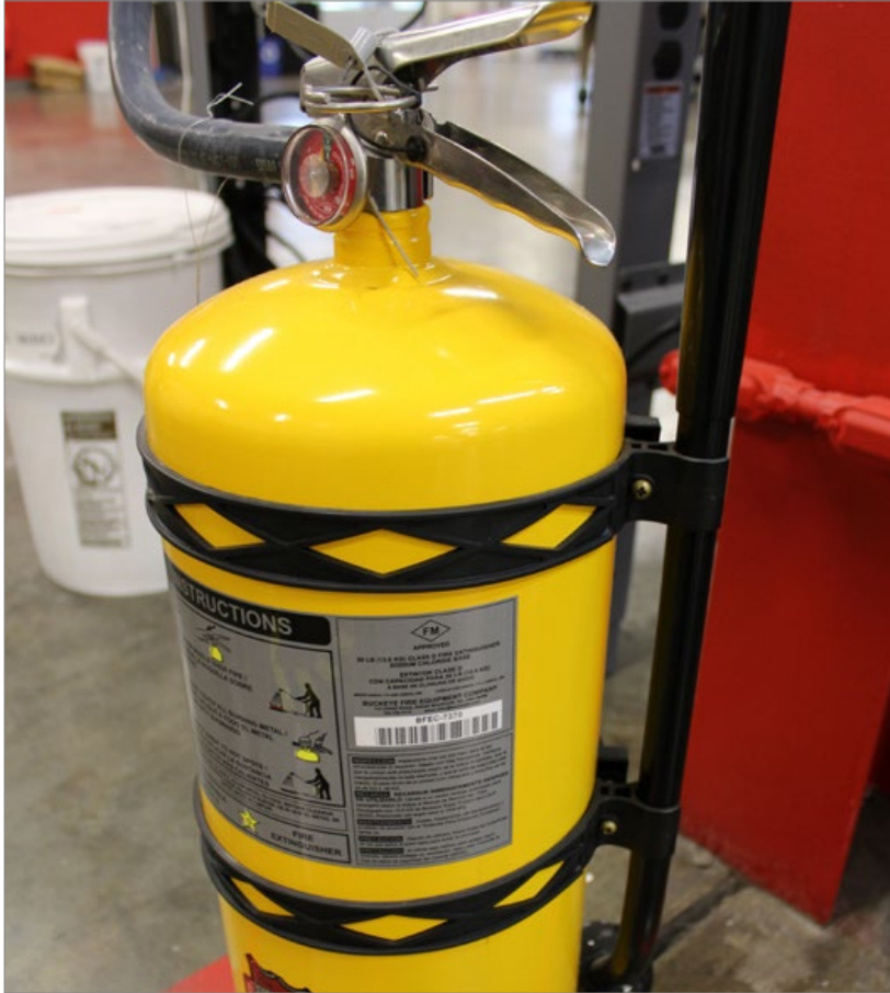
Fig. 4 Metal powder fires must be extinguished using appropriate media. Water-based fire extinguishers, with some materials, have the potential to actually exacerbate a fire caused by metal powders
