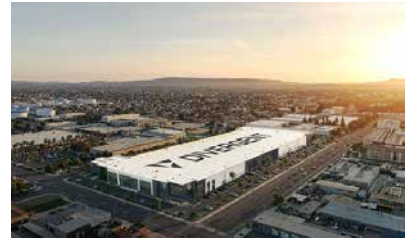
Divergent announced plans to expand its manufacturing operations, with a new 40,000 m 2 facility in Long Beach (Courtesy Divergent Technologies)
