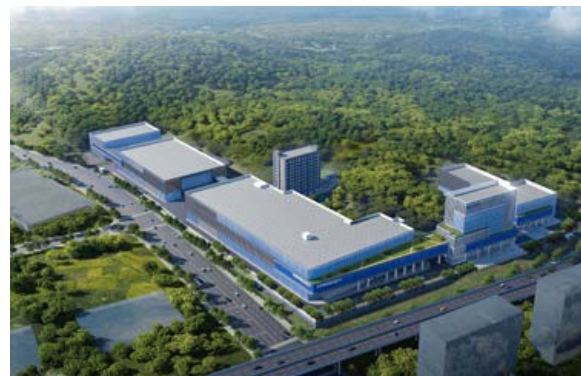
Farsoon's new facility will include 140,000 m 2 of floor space (Courtesy Farsoon)
