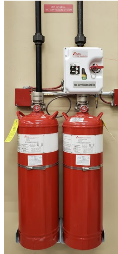
Fig. 6 Dry chemical system actuator and compressed extinguishing agent
