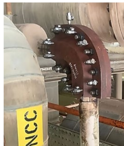
Drawing of the additively manufactured clamp (left) and the final Additively Manufactured clamp installed at a Shell site (Courtesy Shell)
