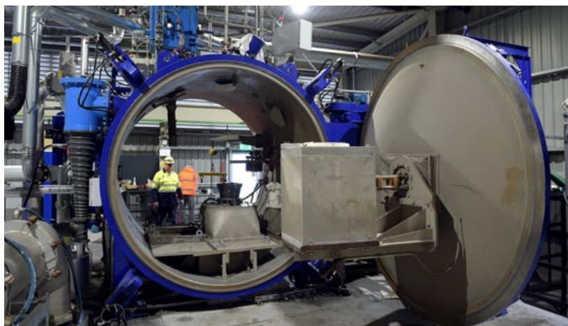
Liberty Powder Metals' Atomiser Plant in Teesside, UK (Courtesy Liberty Powder Metals)
