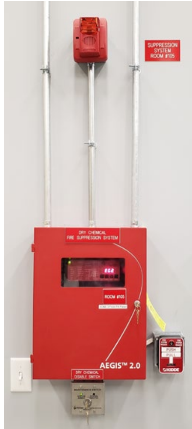
Fig. 5 Dry chemical system controller and communication panel
