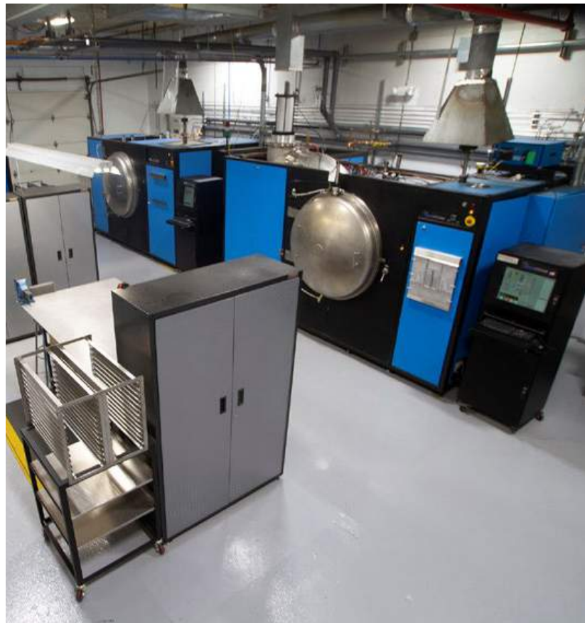
Fig. 3 This view of the DSH facility illustrates how additional facilities required to run a furnace, such as process gas supply, air, power, water cooling systems, etc., involve expenses that can often go unrealised in an analysis
