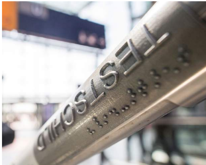
Fig. 6 Handrail produced by metal AM with text in German and braille (Courtesy Deutsche Bahn)
