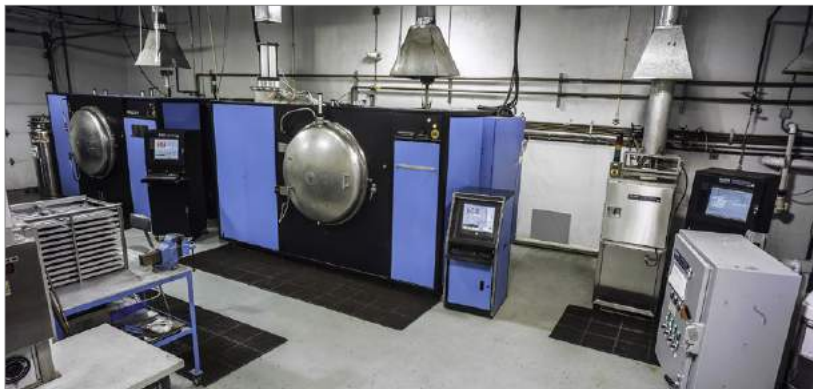
Vacuum debinding and sintering furnaces for MIM and MIM-like processes at Elnik Systems/DSH in Cedar Grove, New Jersey, USA
