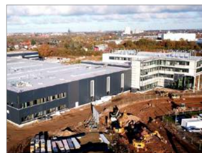
SLM's new headquarters under construction in Lübeck, Germany
