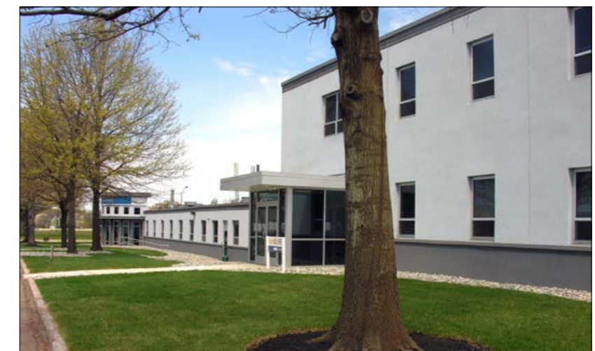
Fig. 1 Exterior view of the Hoeganaes Innovation Center in Cinnaminson, New Jersey
