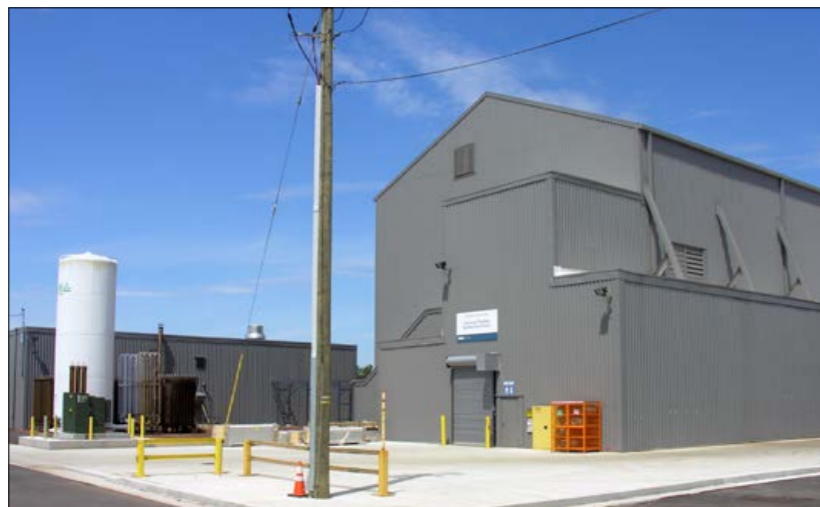
Fig. 2 Production facility at Hoeganaes' Innovation Center
